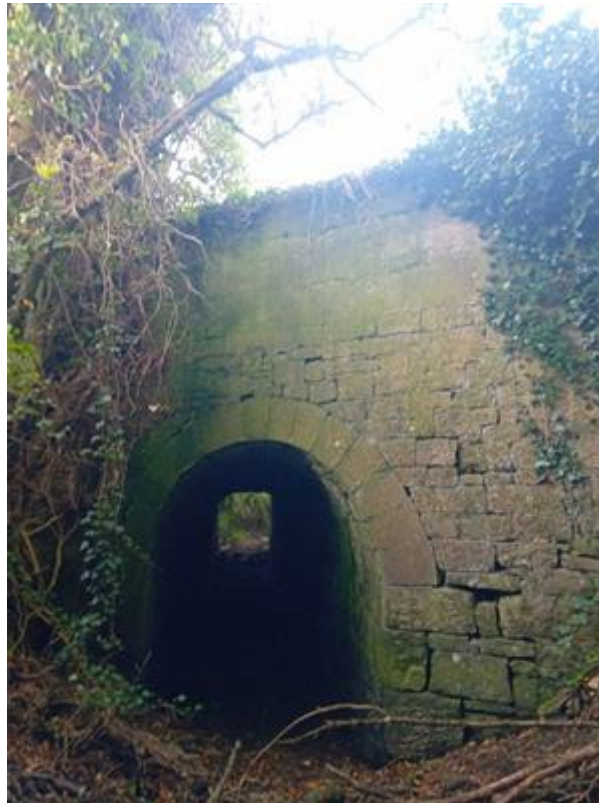
Plate 6-40: Borrisbeg Stream Bridge (2)
