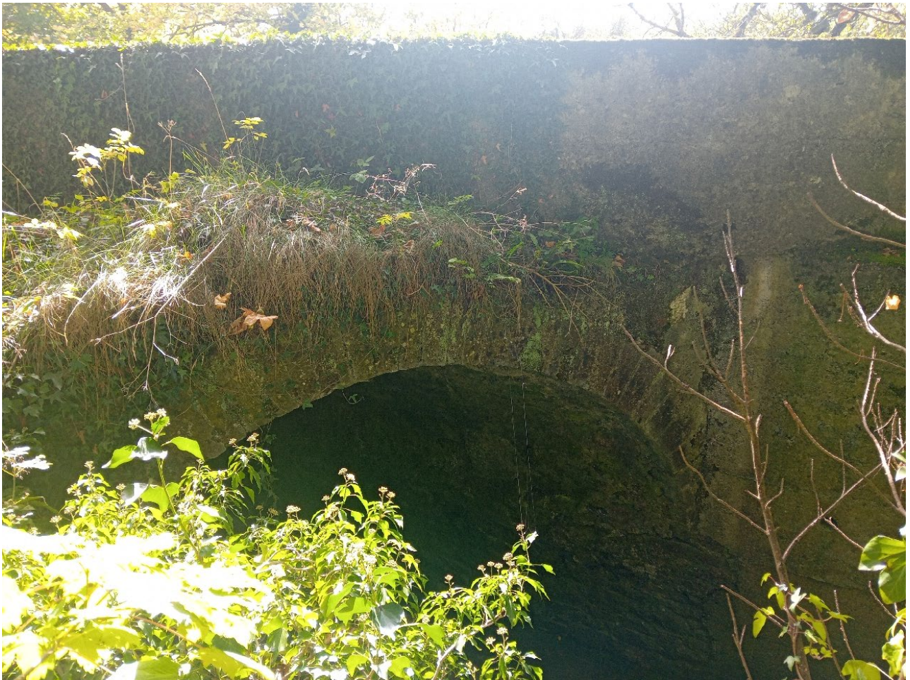
Plate 6-41: Gorteenahilla Stream Bridge (upstream)
