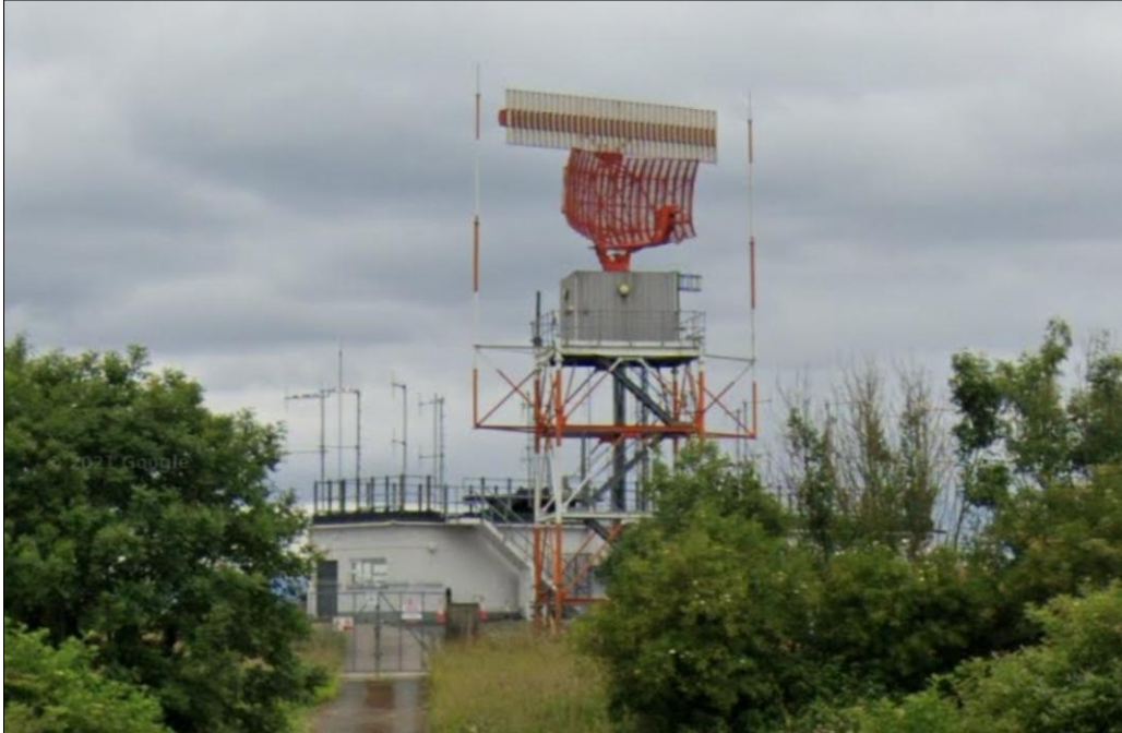
Figure 11. Dublin Airport MSSR Radar Station #1
