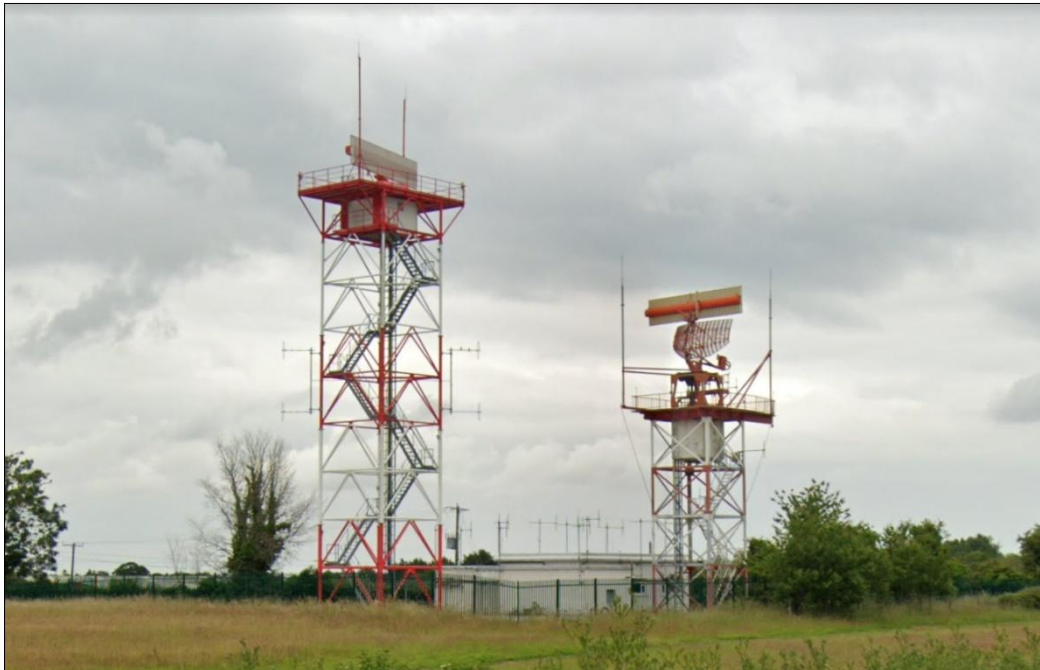
Figure 12. Dublin Airport MSSR Radar Station #2
