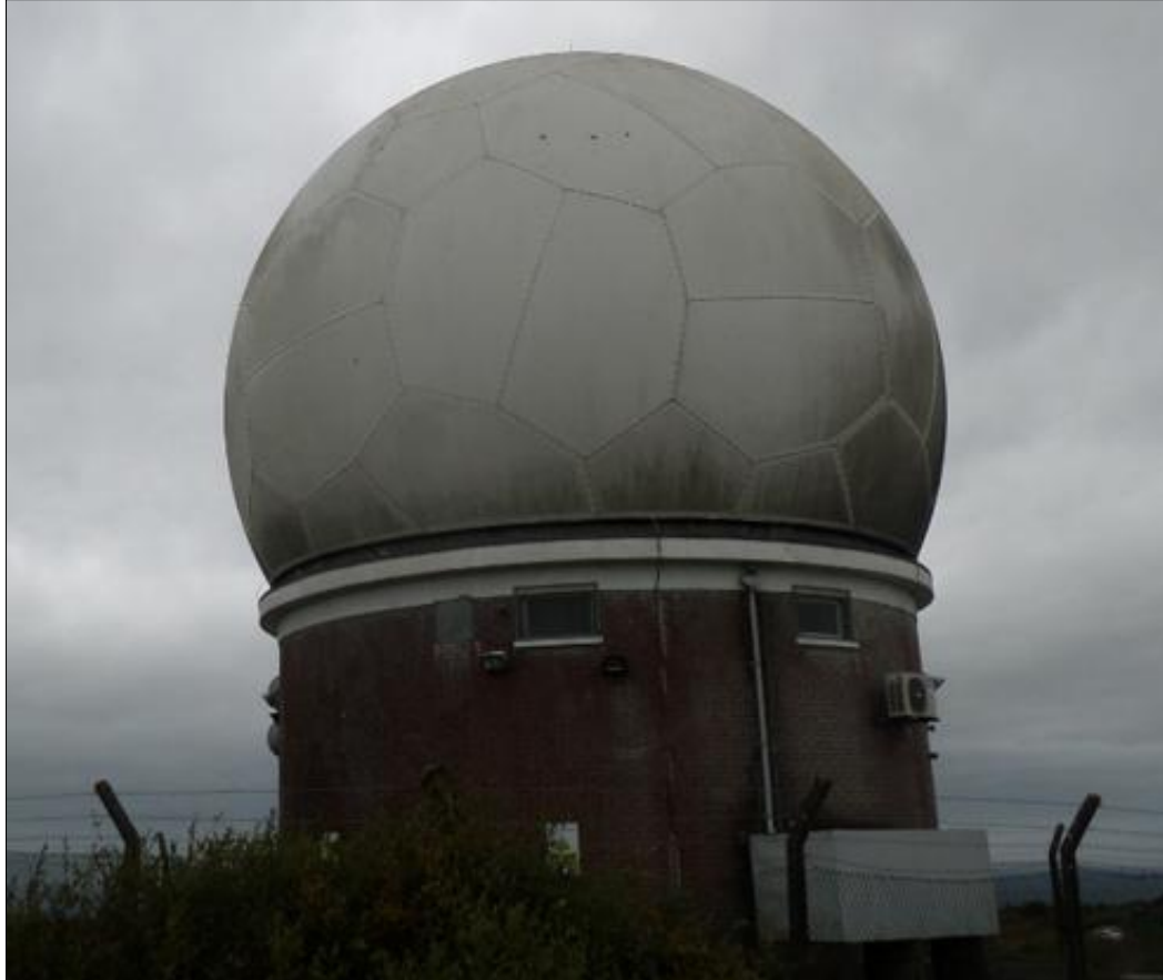
Figure 10. Woodcock Hill Radar Station
