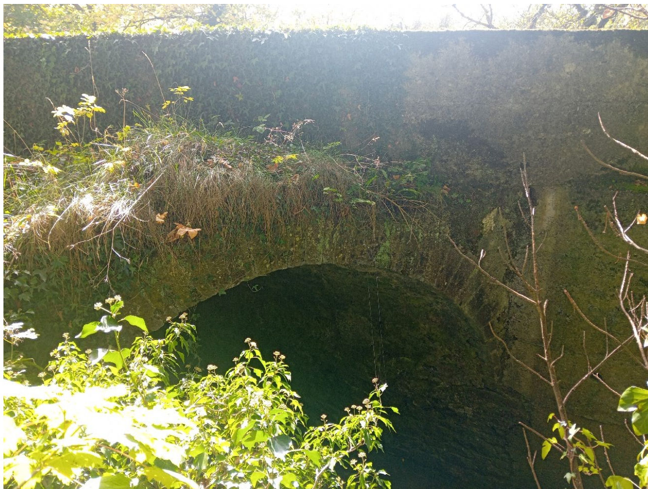
Plate 3-6: Gorteenahilla Stream Bridge (upstream)
