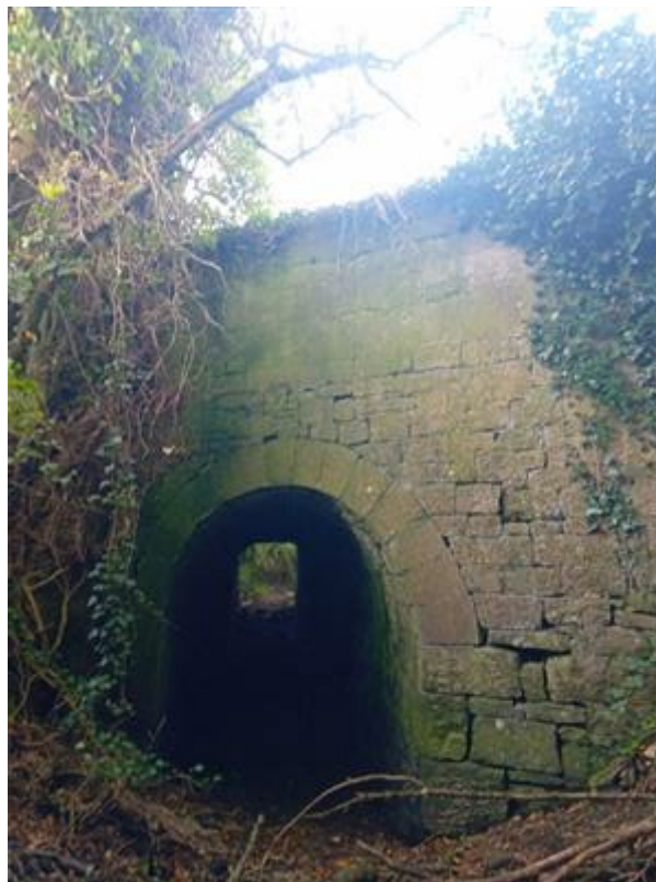
Plate 3-5: Borrisbeg Stream Bridge (2)
