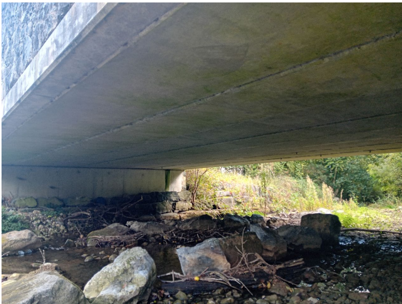
Plate 3-10: Lisdowney Stream Bridge
