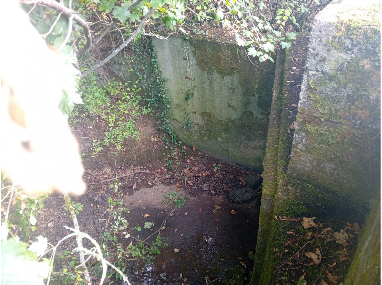
Plate 3-9: Lismaine Stream Bridge
