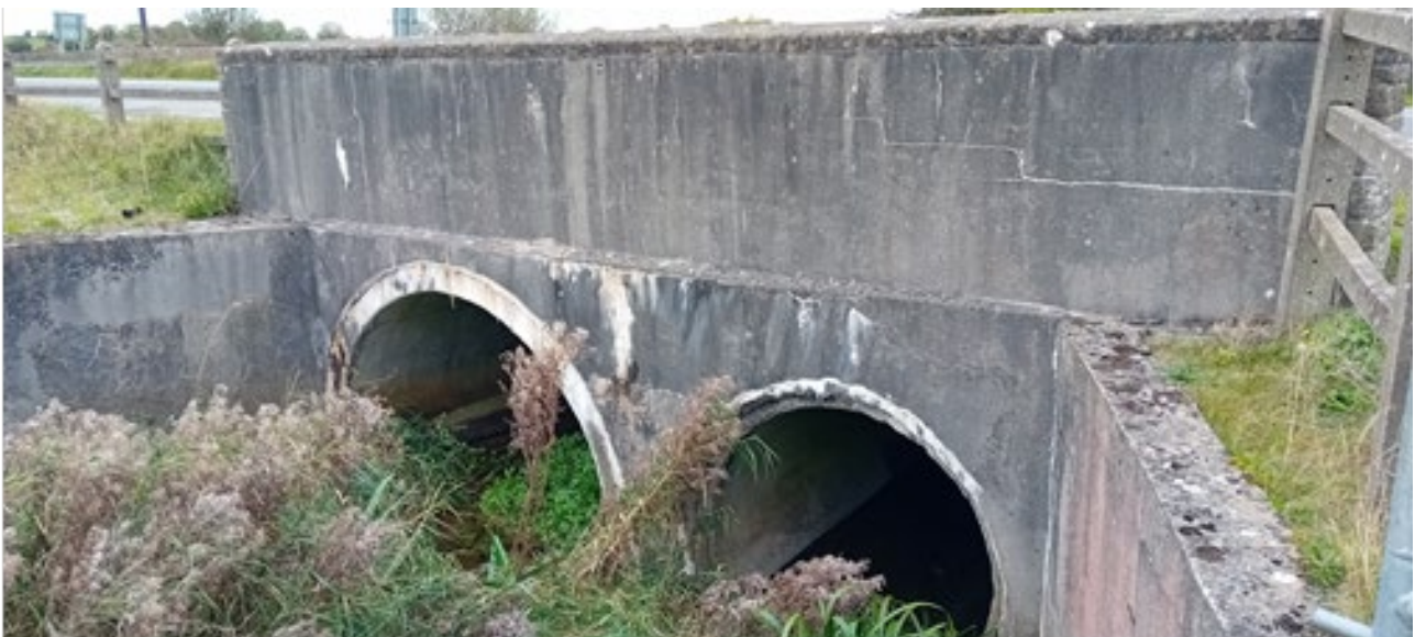
Plate 3-2: Goul River Bridge
