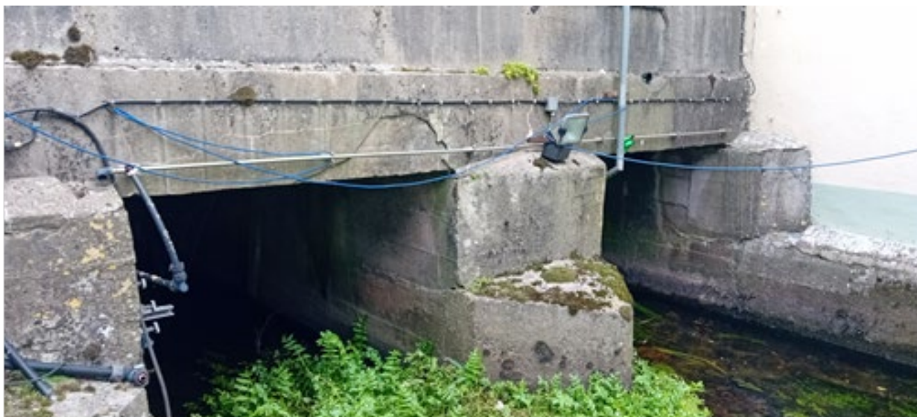
Plate 3-3: Aldreagh Stream Bridge
