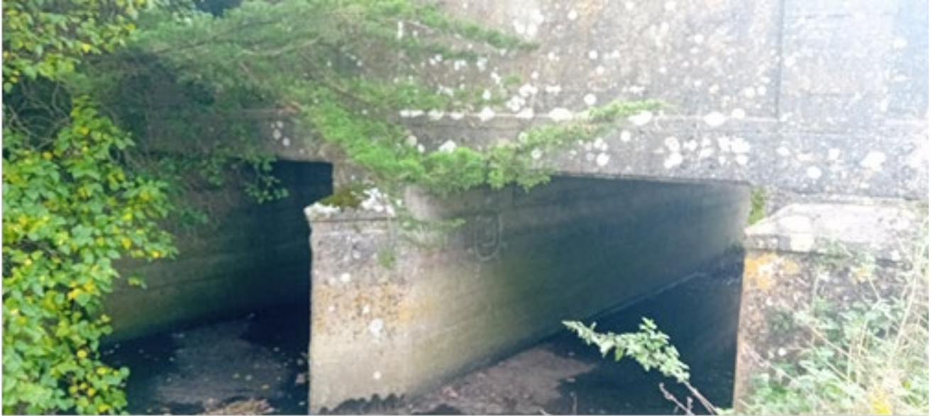
Plate 3-1: Black River Bridge
