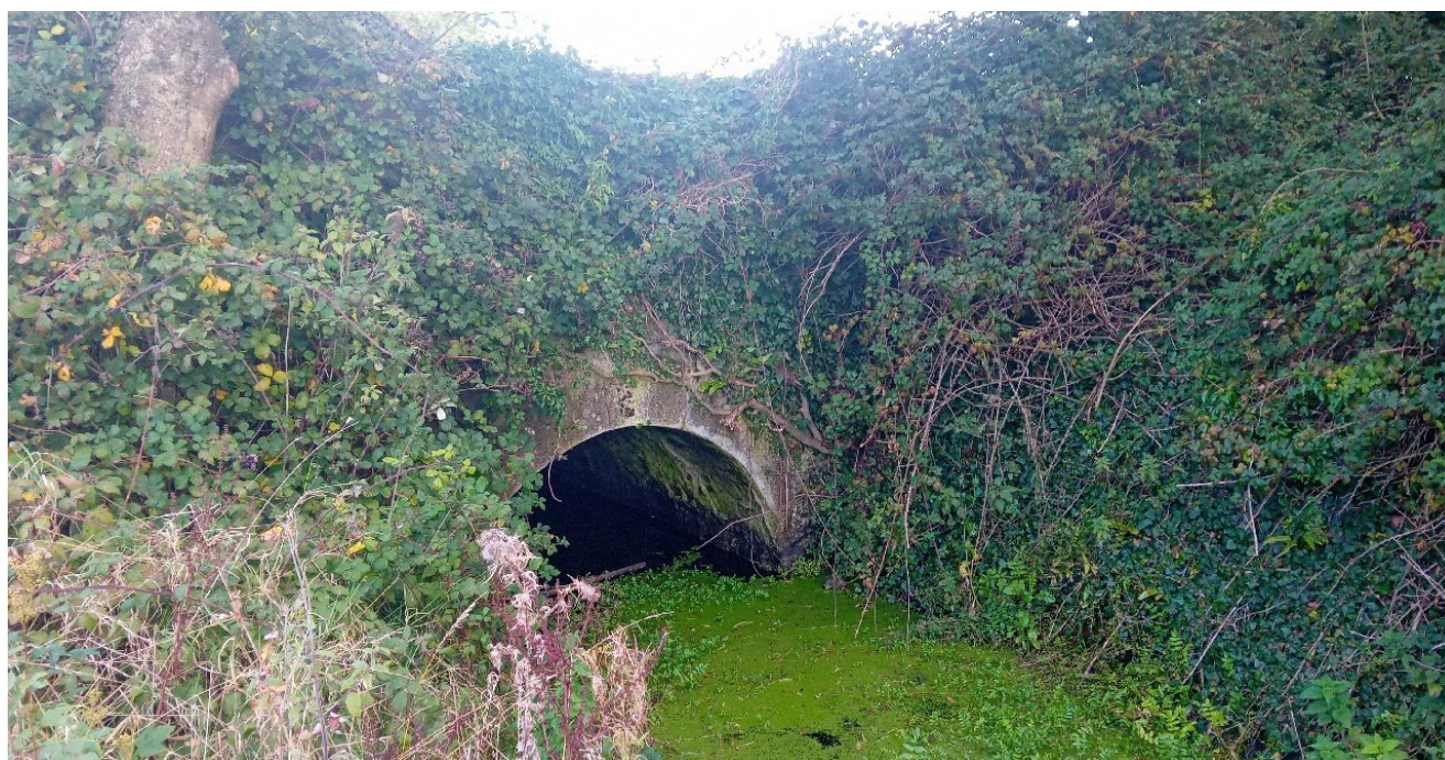
Plate 3-4: Borrisbeg Stream Bridge (1)
