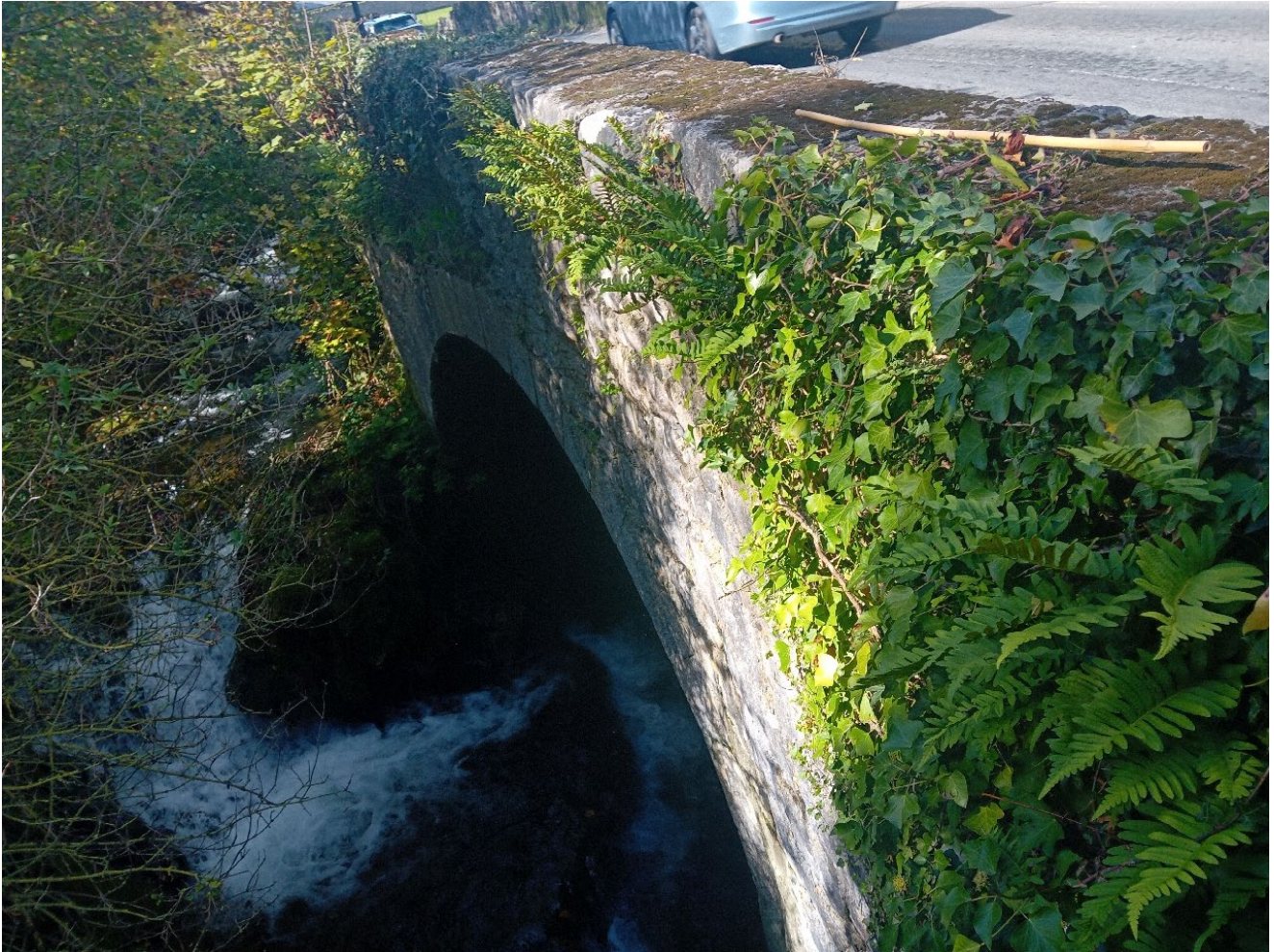
Plate 3-7: Gorteenahilla Stream Bridge (downstream)
