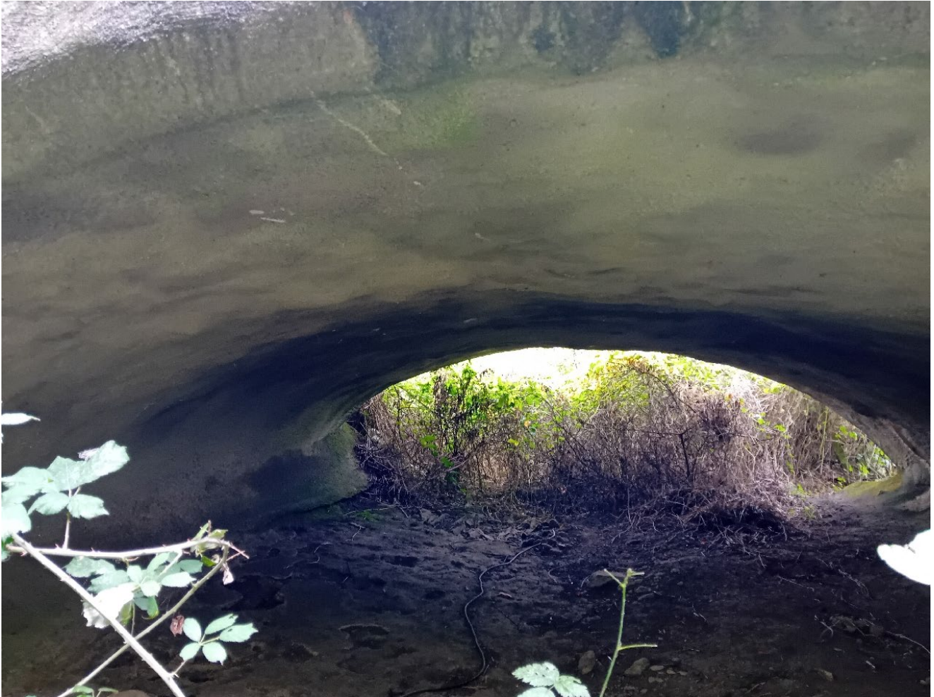
Plate 3-8: Bridge over un-named channel on northern outskirts of Freshford
